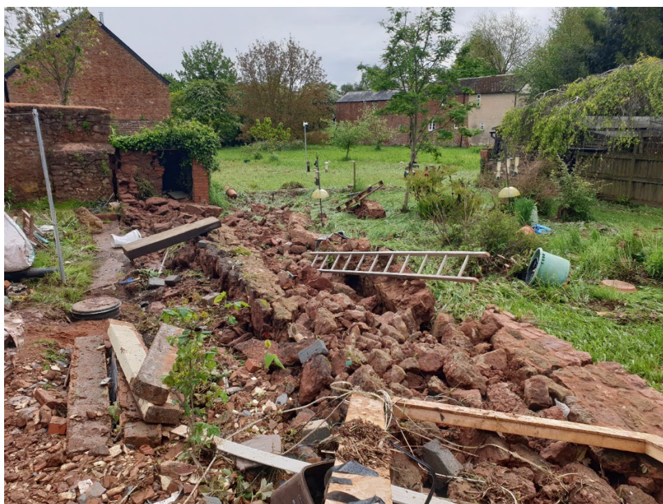
Figure 1. Flood Damage, Milverton, May 2023
